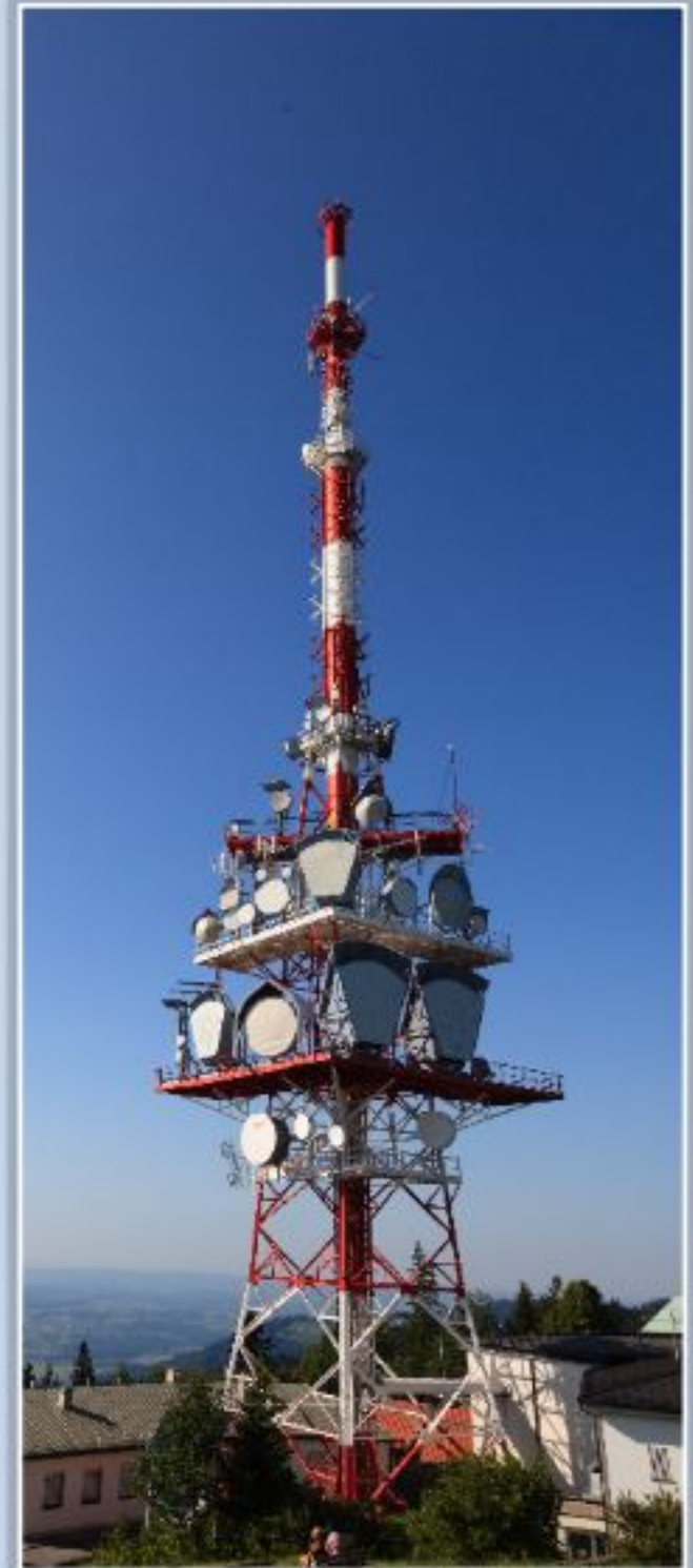
Austrian telecom tower.
